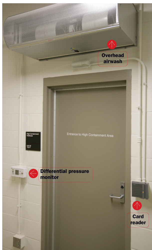
FIGURE 3. Containment Entry Vestibule with Overhead Airwash, Card Reader, and Differential Pressure Monitor*
